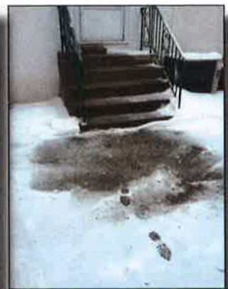
Anti-icing application vs. No application
